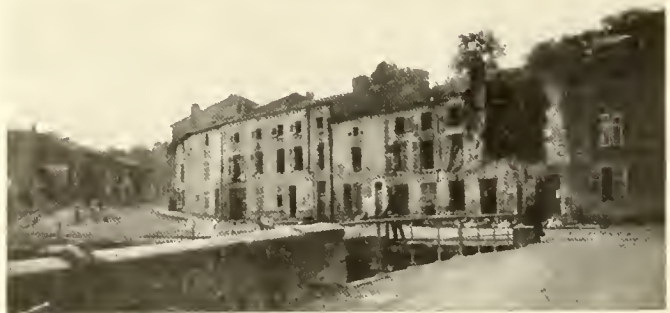
Traffic bridge in the center of the town which was a special artillery target.
